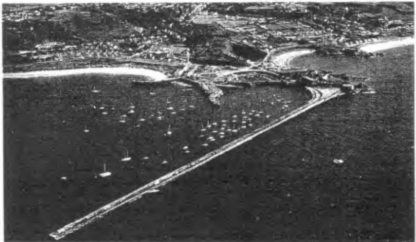
Plate 1 The existing Admiralty Breakwater
