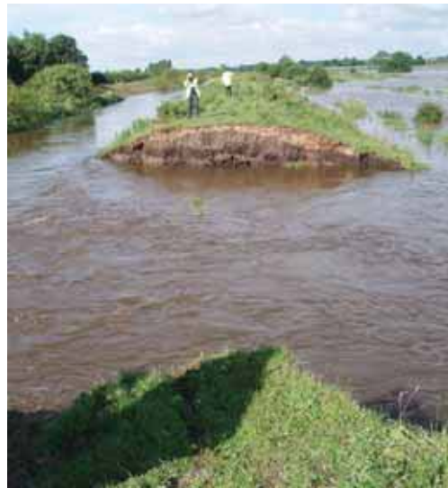
Figure 4. Breach at Auckley during Summer 2007 floods.
